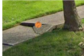
Figure 1: An example of labeling a surface problem. Figure 2: Common high severity surface problem in Oradell.
