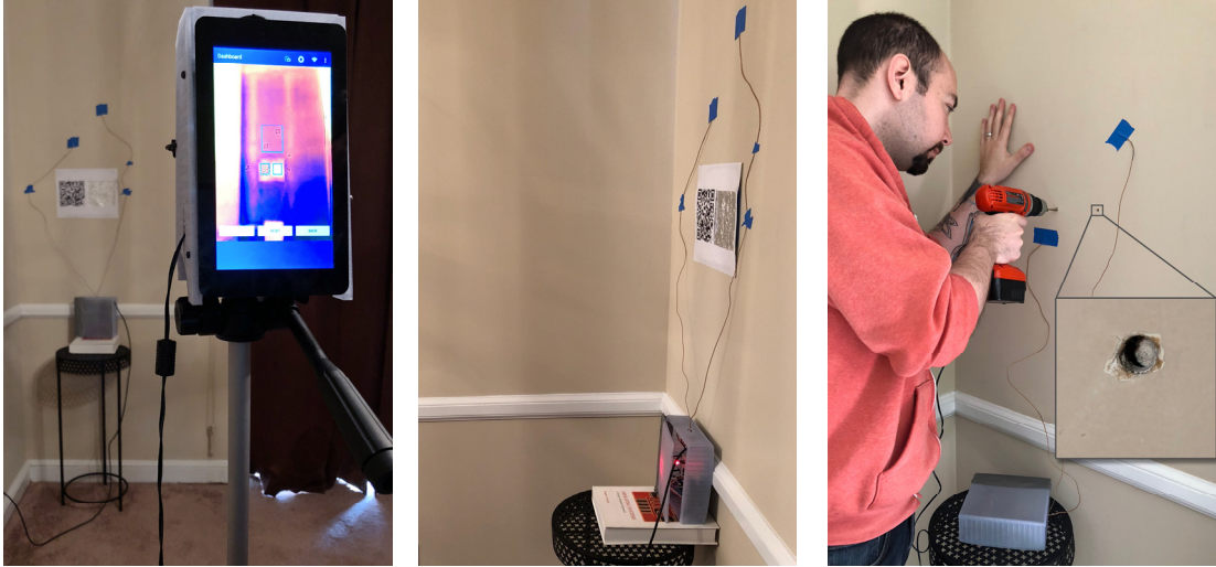
Figure 7.6: Deployment setup for the validation experiments. The sensor system in the process of being configured (left) to analyze the area framed by the thermocouples (middle), and destructive testing to verify composition of wall assembly (right).
