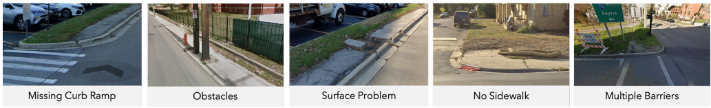
Figure 1. Examples of sidewalk accessibility barriers. The last sub-figure shows multiple barriers present together: missing ramp, no sidewalk, and uneven surface. Images from Project Sidewalk [78].
